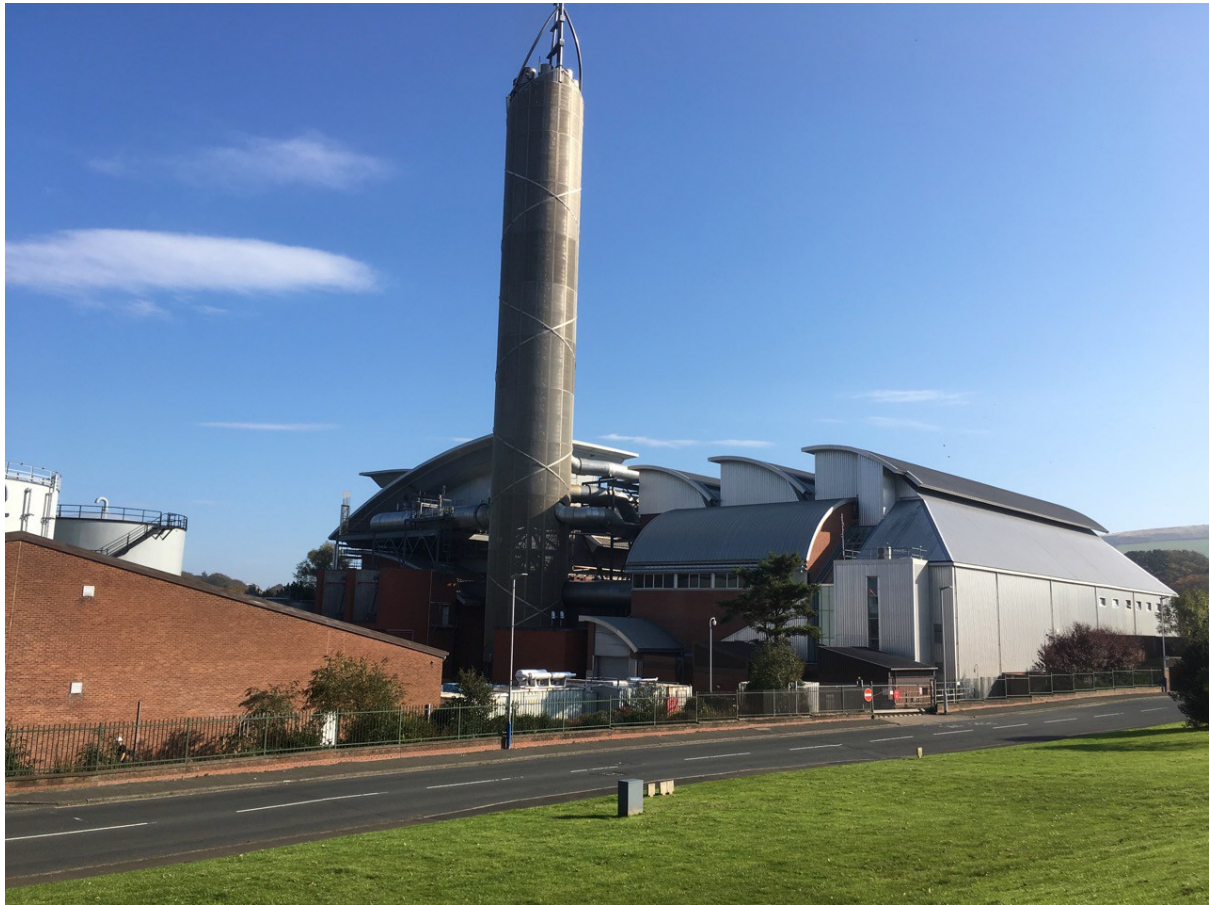
Gas turbine electricity generating plant, Pulrose, Isle of Man
